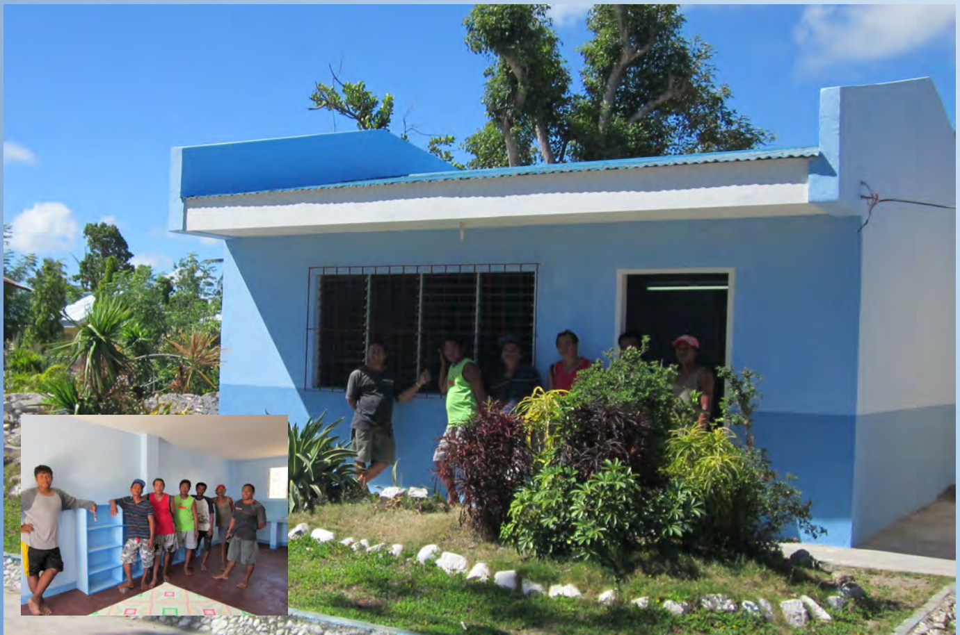
The first SPED Center to be completed: Students with disabilities in Carles, Iloilo will be served by the Center.
